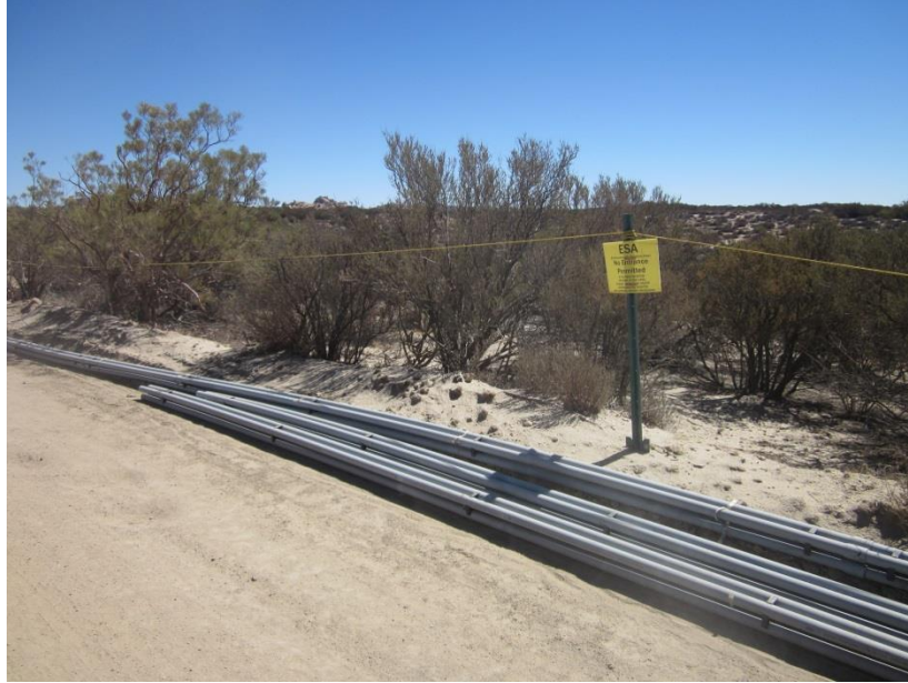
Photo 1: In accordance with MM-BIO-1c and MM-BIO-1a, biological monitors were onsite to ensure construction remained within the approved work limits.
